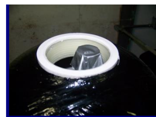
Figure 8: How to Block Distributer Tube
