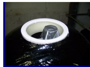
Figure 8: How to Block Distributer Tube
