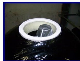
Figure 8: How to Block Distributer Tube
