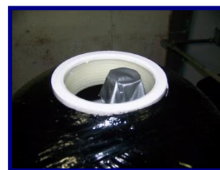
Figure 8: How to Block Distributer Tube
