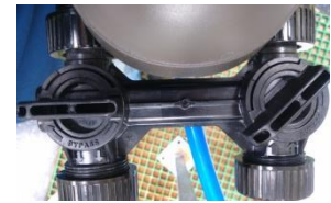
Figure 14: Opening bypass valve's inlet
