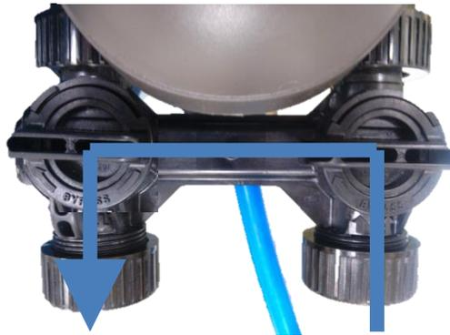
Figure 18: Bypass Operation
