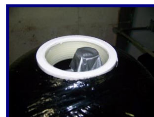
Figure 9: How to Block Distributer Tube
