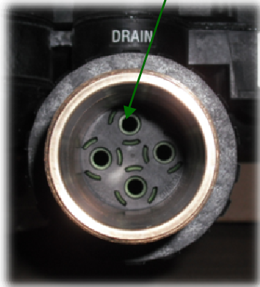
Drain Line Flow Control *Installed CORRECT Buttons On Inside.
